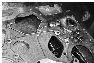
Fig 5-24 Lubricating Pipes Installation
